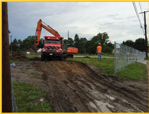
Sorority Housing Construction Day One July 2015
