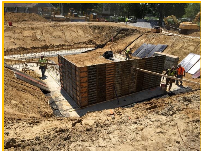
Sorority Housing Construction Day 18 July 2015
